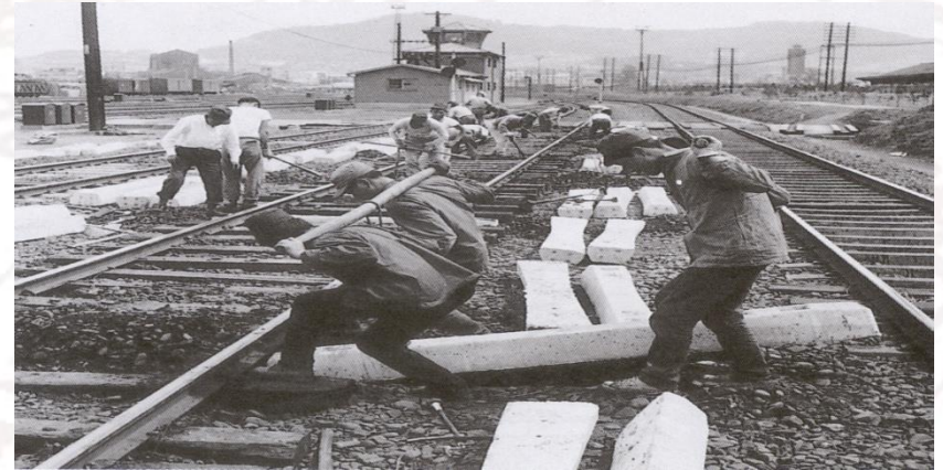
Railroad construction sites
